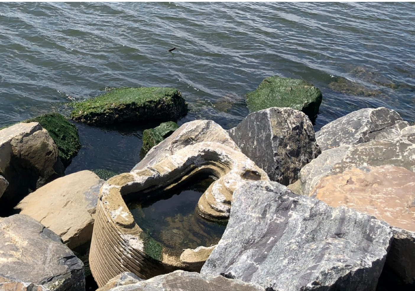
The breakwaters are designed to foster biodiversity for a range of species incorporating a wide range of habitat-supporting features.
